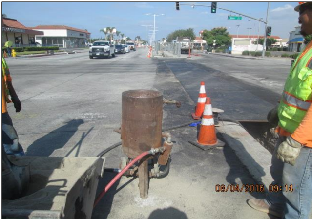
Tank for Supplying Sand to Fill Void in Sleeve
