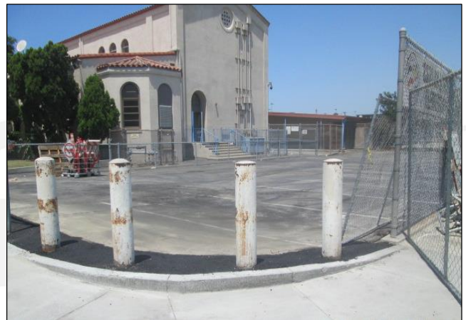
Looking to Parking Lot from ADA Ramp West of Orrick
