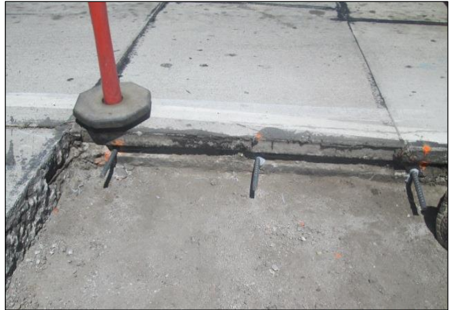
Dowels at Approximately West of Main St.
