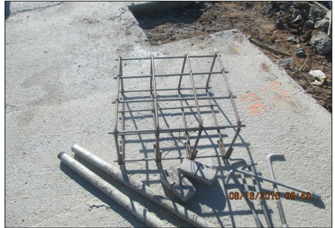
Modified Rebar Cage for F-1 Light Foundation
