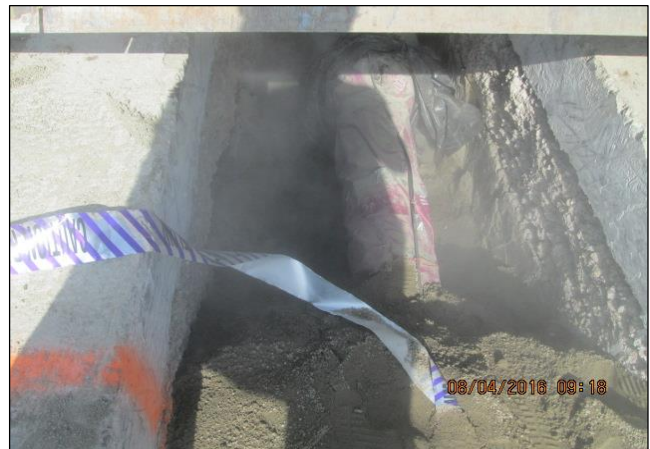
Sleeve Being Sand Filled
