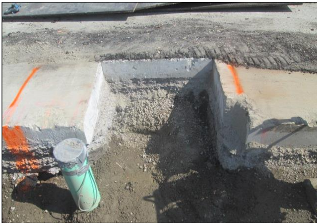
Painted Area to be Removed in Compliance
