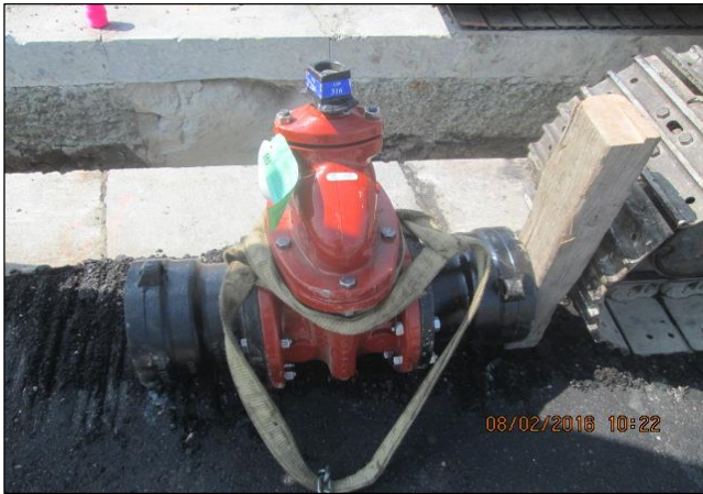
Recycled Water Gate Valve Being Installed
