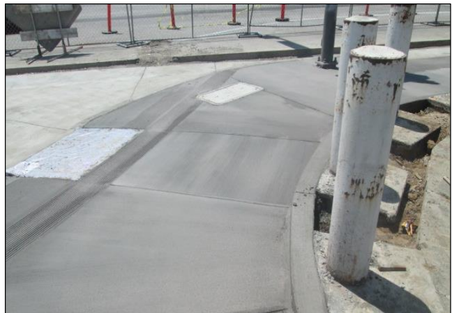
ADA Ramp at Carson Elementary
