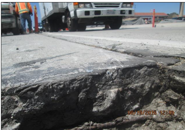
Rebar Existing in Existing Pavement Station West of Main St.
