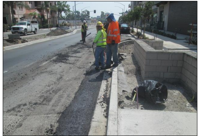
Twelve Inch Silver Asphalt Concrete Fill
