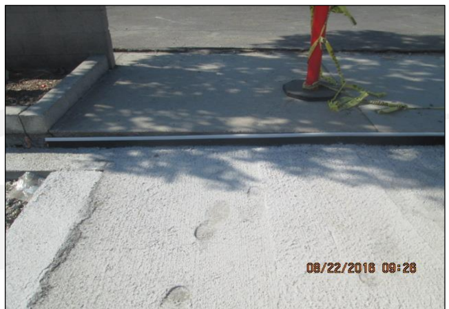
Expansion Backer Between Pavers and Sidewalk
