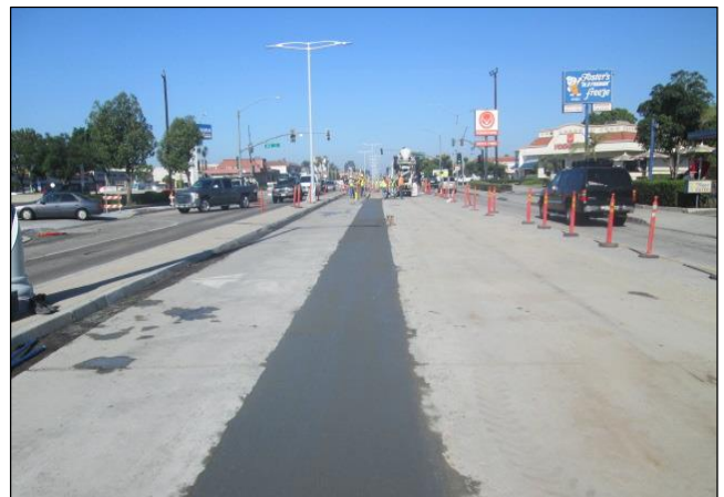
High Early Portland Cement Concrete on Carson at Main
