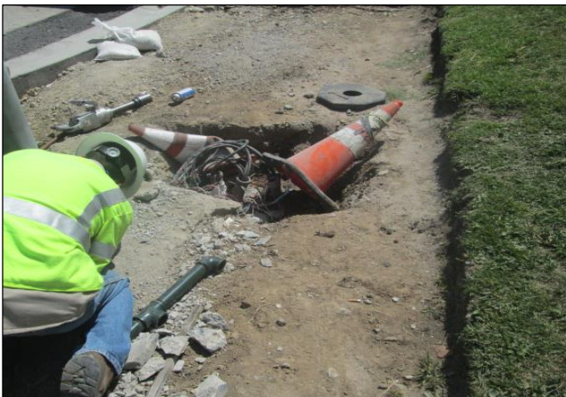
Belco to Provide Pull Box at Orrick Traffic Light
