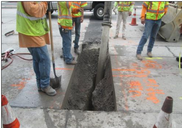
Ongoing Pot Holing Southbound Main at Carson
