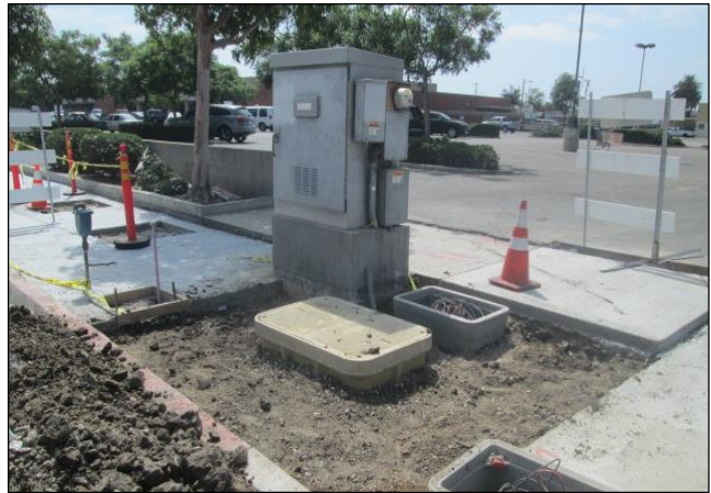
Main St. Southeast Corner Electrical Box
