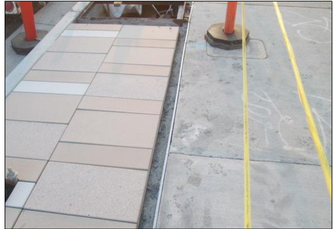
3" Gap Between Pavers and Sidewalk
