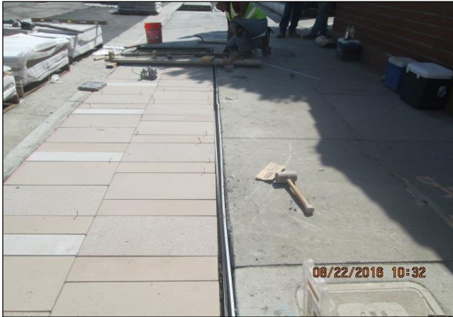
1" Strip Left Between Pavers and Sidewalk
