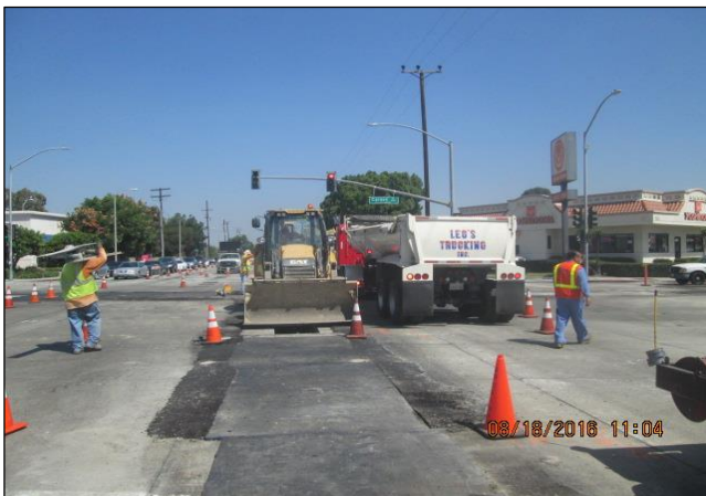
Main Street Northbound Trench line for Recycled Water Line
