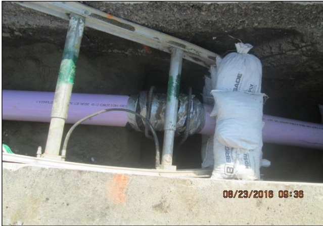
Recycled Water 22 Deg El Ready for Thrust Block
