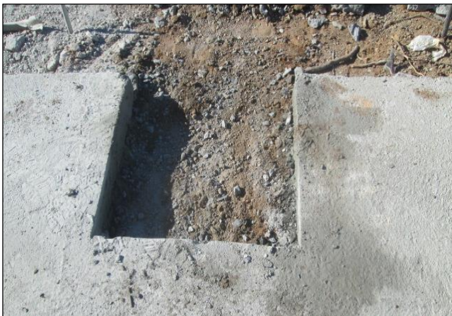
Ready for F-1 Light Foundation
