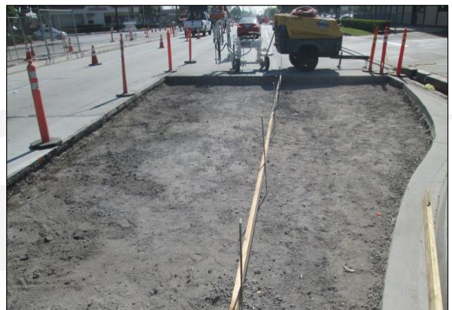
Right Turn Lane for Going Southbound on Main Ready for Dowels
