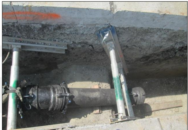
Recycled Water Passing Over Oil Lines
