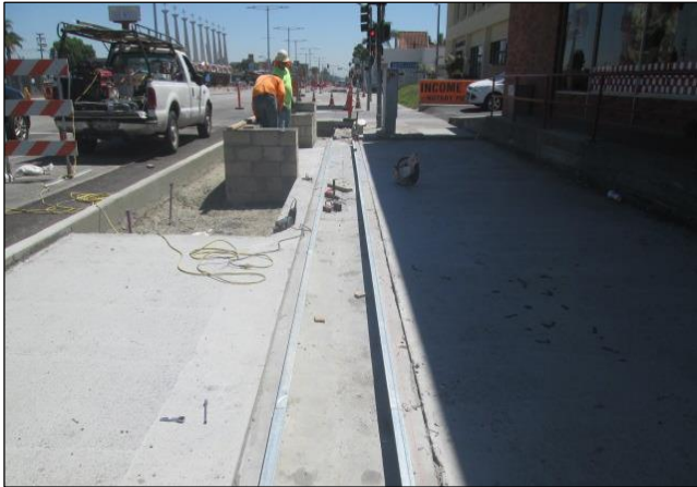
Angle Iron Rail for Grating
