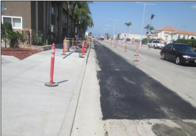
Paving West of Moneta
