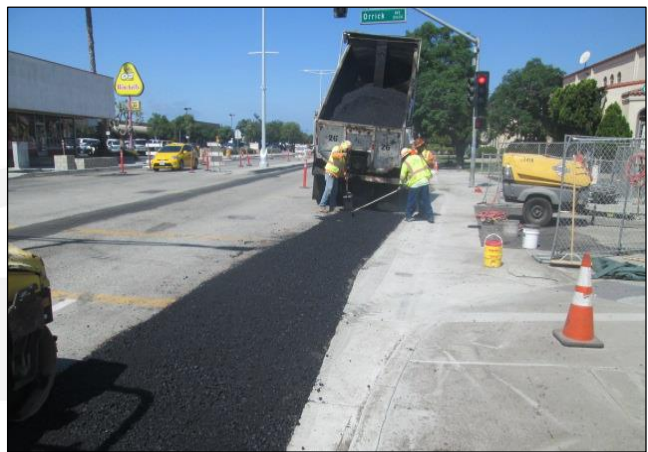
Paving Slot at Orrick and Carson Elementary School
