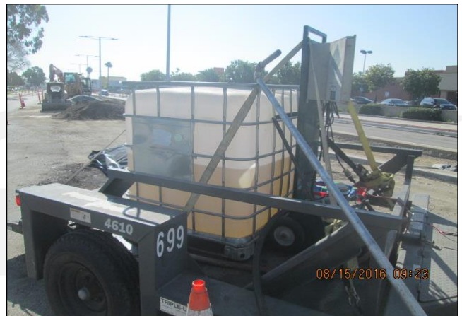
Concrete Admixtures for Portland Cement Concrete on Carson and Main
