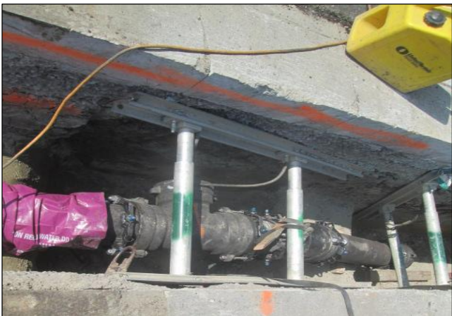
Recycled Water at Main Street Intersection Tee Going South
