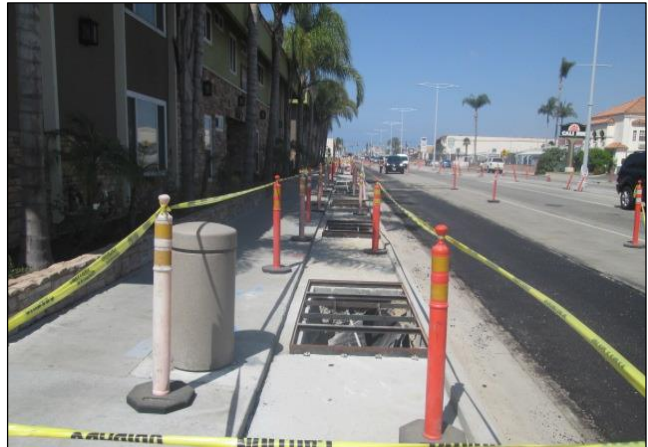
Tree Wells Have Been Taped Off
