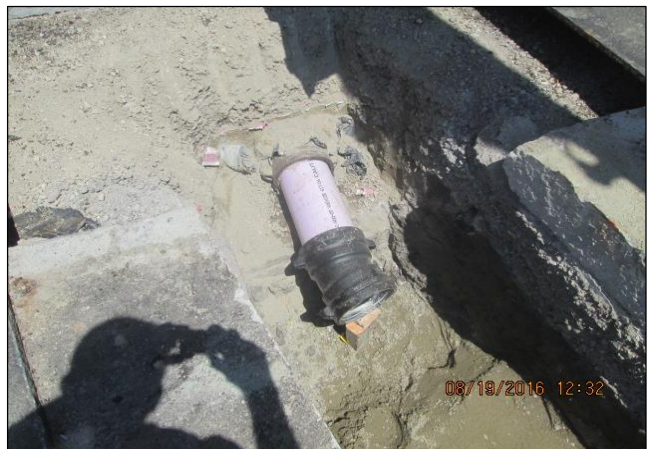
10" Stick of Recycled Water Line in Trench Southbound on Main
