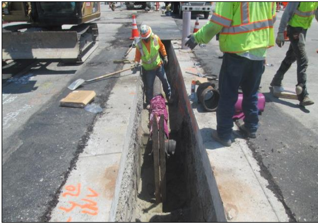
Ductile Iron Recycled Water with Tee Going South
