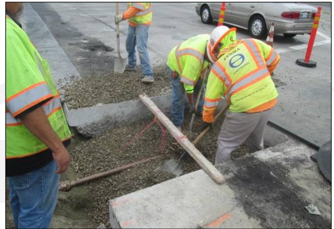
Placing Rock in Area of the Air Vac Main Intersection
