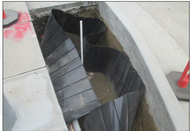
Root Barrier Prior to Planting
