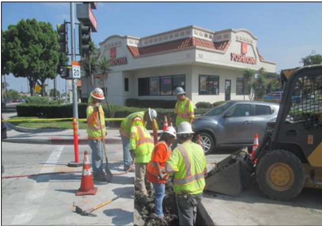
Trench for Air Vac at Main and Carson
