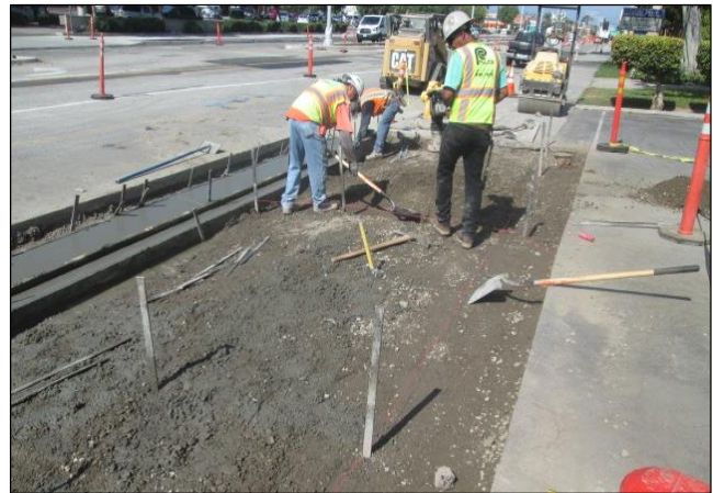
Second Driveway at Elementary School
