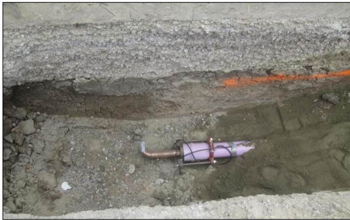
Blow Off at Termination of Recycled Water Line
