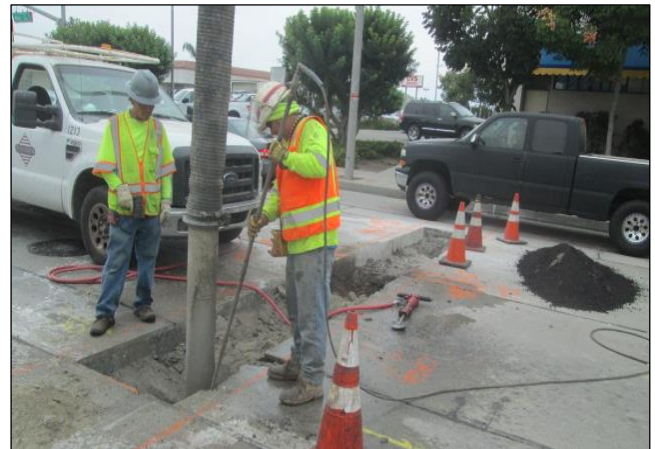
Pot Holding Operation on Southbound Main North of Carson
