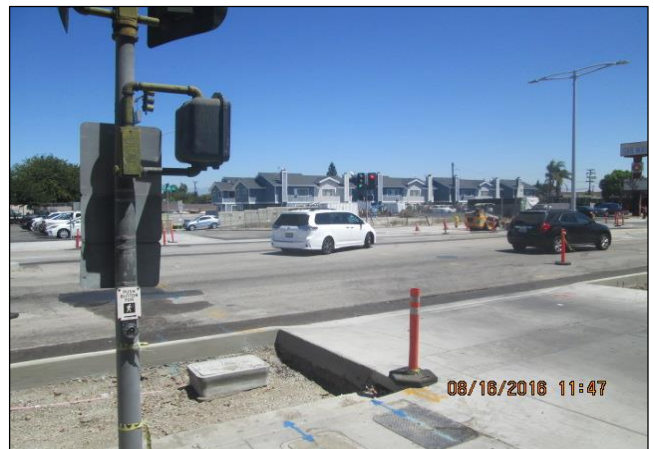
Drive to Rear of Winchell's Treated as a Street Crossing
