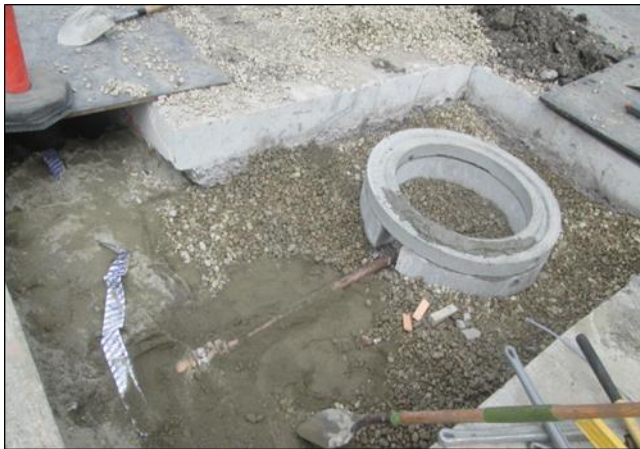
Air Vac Man Hole Center of Carson at Main
