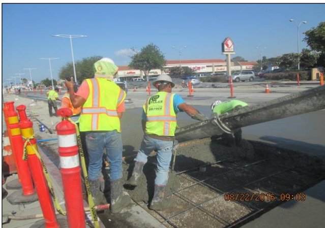
Placing Right Turn Lane at Carson and Main
