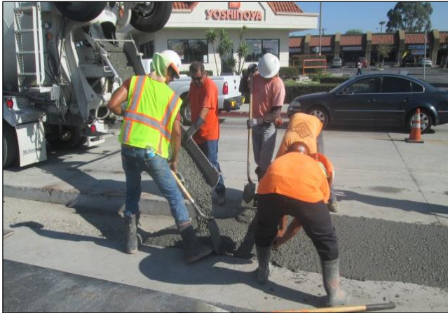
High Early Portland Cement Concrete on Carson at Main
