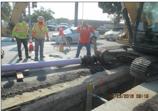
Length of 8" Recycled Water Line with Ball Valve Lowering into Trench
