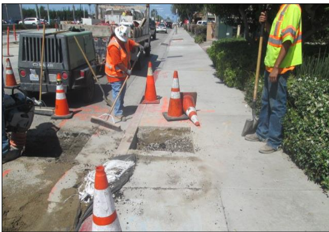
Location for Blowoff Assembly/ Recycled Water Line End West of Main St.
